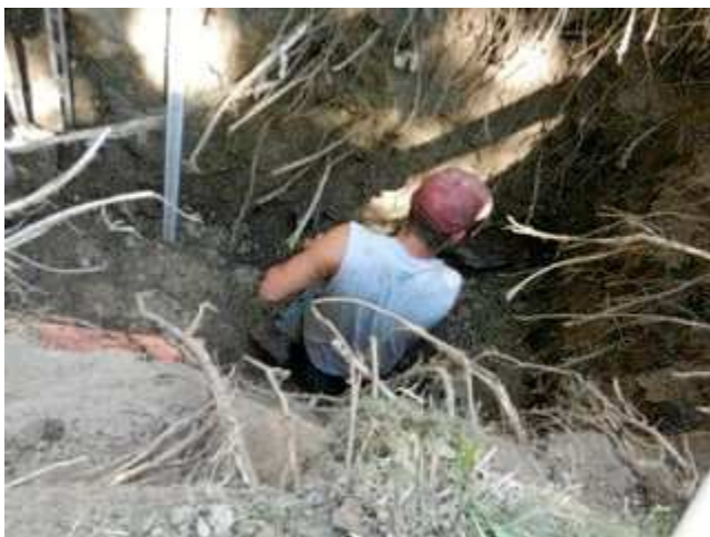
A PVC pipe from the sidewalk drain and the pipe that was bored were connected.
