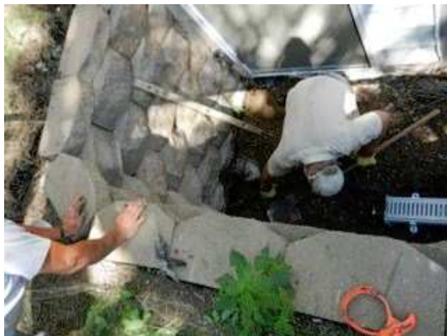
The cement workers and the excavator workers dug a trench from each side under the wall.
